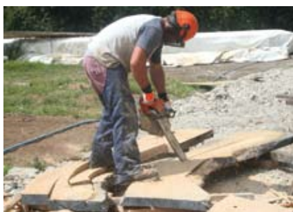
Cutting oak frames with a chain saw
